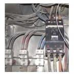
Bad electrical connections due to any loose or corroded terminations which can generate heat. Measuring temperature with a safe, noncontact infrared thermometer will help to identify any trouble spots.
